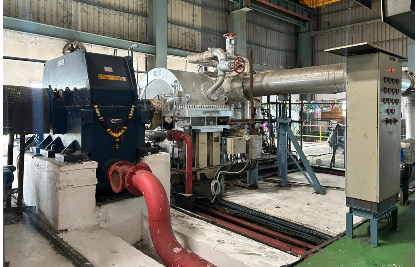
Picture 4: (a) Boiler produce steam that's used in many stages of sugar manufacturing, (b) Turbine section generate electricity and power for the plant's uses and export
