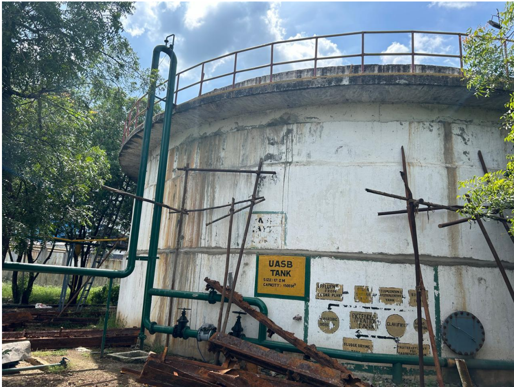
Picture 6: (a) UASB (Anaerobic) Reactor and (b) Aerobic treatment of wastewater
