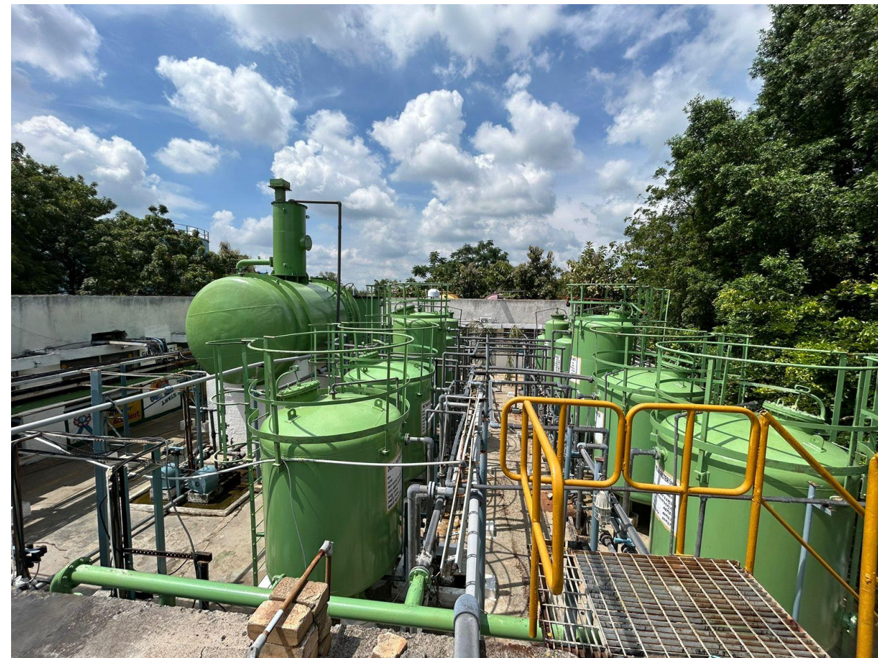
Picture 5: (a) Water treatment plant capacity of 25 m 3 /hr and (b) WTP analysis Lab
