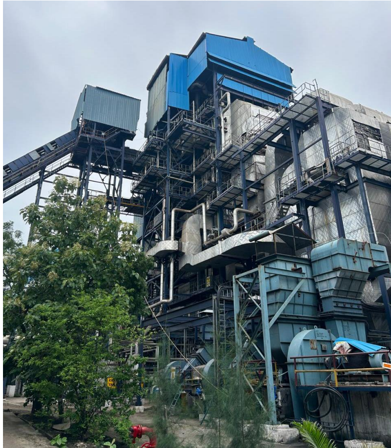
Picture 4: (a) Boiler produce steam that's used in many stages of sugar manufacturing, (b) Turbine section generate electricity and power for the plant's uses and export
